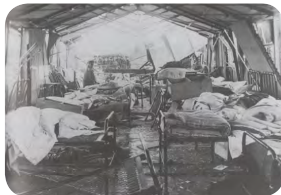
A bombed ward in the Hospital at Etaples, May 1918.
