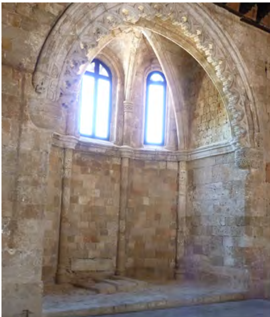
In the centre of the ward is an alcove which was originally a chapel. Most mediaeval hospital wards had facilities for saying Mass.
