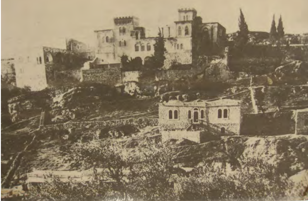
The building in the foreground is the 'first' St John Ophthalmic Hospital, Jerusalem, 1890, eight years after its establishment.
