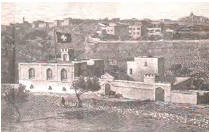
The Hospital as seen from the hill on the western side of its Bethlehem Road frontage, 1894. Beyond the building is the Valley of Hinnom and Mount Zion and the Old City of Jerusalem above the valley. This pencil drawing of the Hospital seems accurate in its detail by comparison with contemporary photographs. (Image from the Hospital's Annual Report for 1894.)
