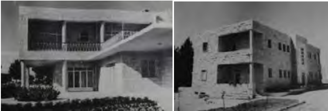
The Warden's House and Nursing Sisters' Home (1960). 29
