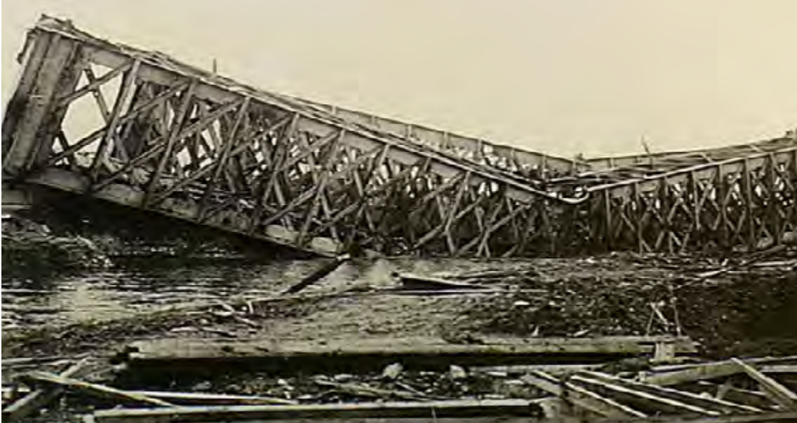
A railway bridge across the Somme destroyed by German shelling in 1918. Captain Owen B Williams won his Military Cross for continuing his inspection of the bridge as the shells were exploding around him. Australian War Memorial photograph no. H09074.
