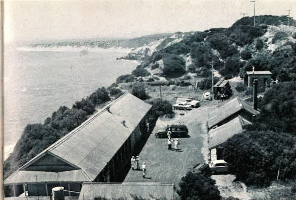
Group of buildings at Officers Training School, Portsea, suitable for use as improvised emergency field hospitals.
